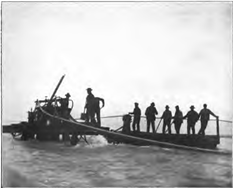
(b) Caisson in Place Over Pipe, Caisson Workers are Placing Concrete.
